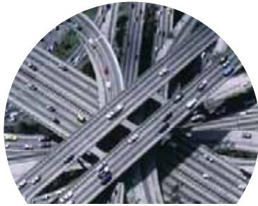
HIGHWAYS AND TRANSPORT
